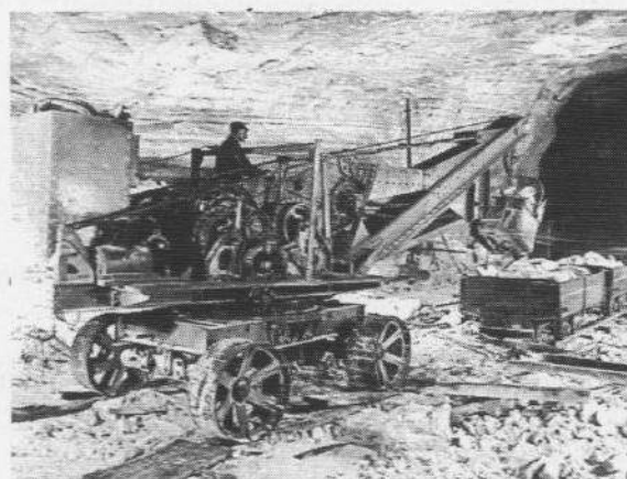
Figure 1. Steam shovel on wood rails. (c. 1912)
